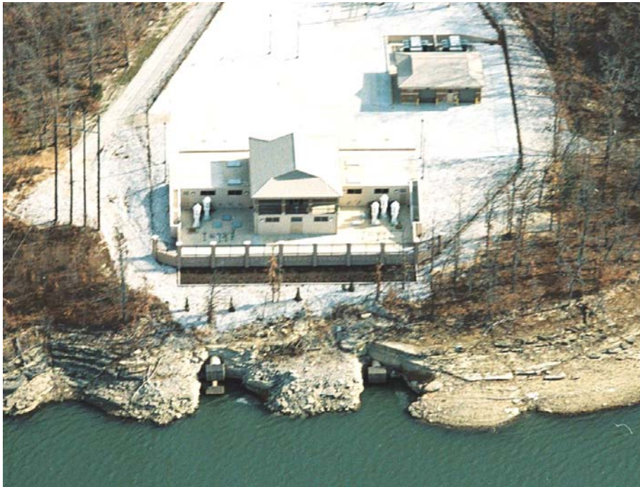
Beaver Water District's new raw water intake
